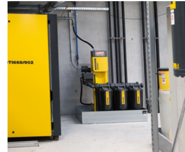
The new AQUAMAT i.CF is the first intelligent oil-water separator.
